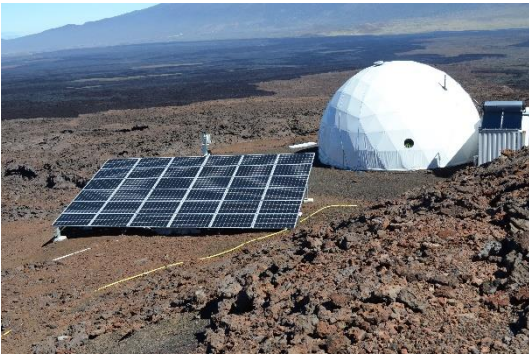
Fig. 1. HI-SEAS habitat with 10kW solar array and water heater with tank. Photo credit: Ansley Barnard.
