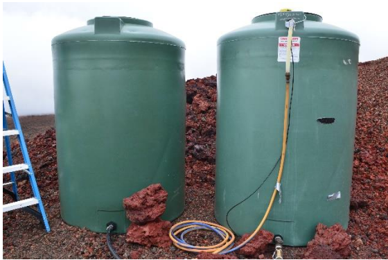
Fig. 5. HI-SEAS external water tanks containing 3785 L (1000 gal) of water. Photo credit: Ansley Barnard.
