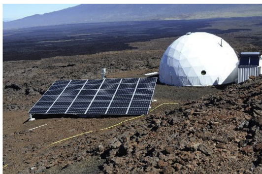
Fig. 1. HI-SEAS habitat with 10-kW solar array and solar water heater with tank. Photo credit: Ansley Barnard.
