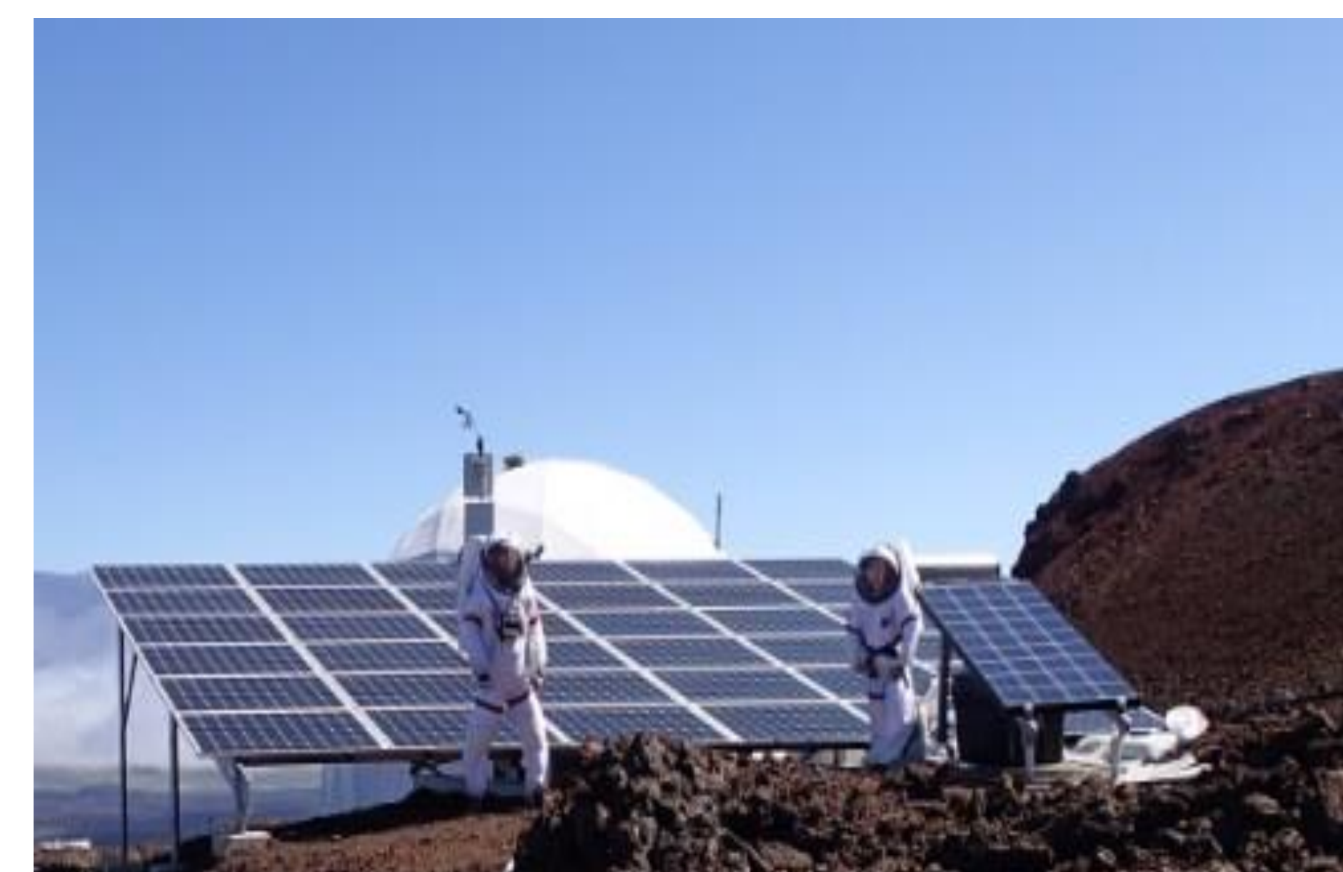
Above: Solar panels during HI-SEAS Mission 2.
