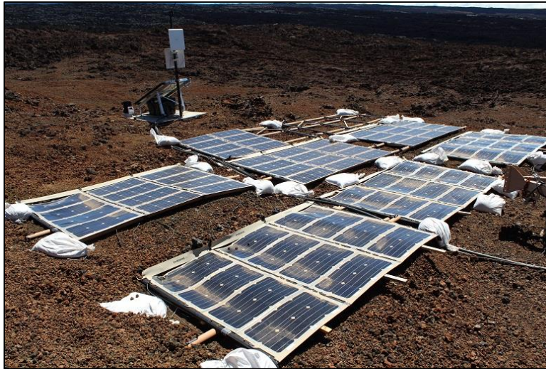
Figure 8 Solar panels provided potential voltage power to the hybrid generator. Photo Credit: Simon Engler
